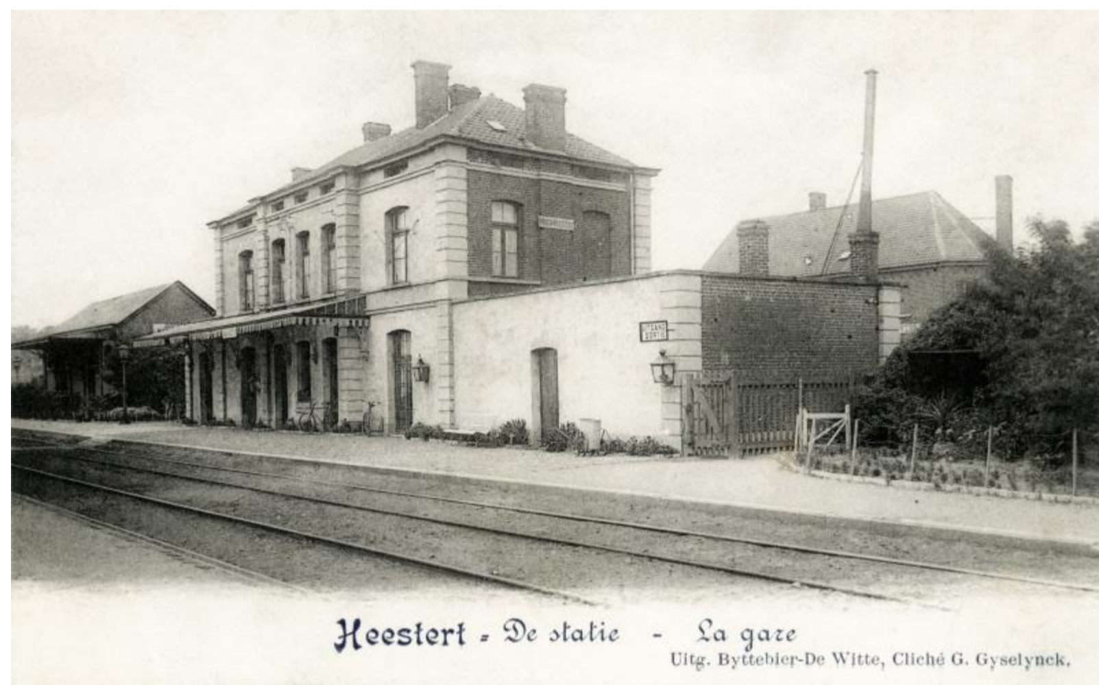
Gare de Moen-Heestert - Moen-Heestert station
